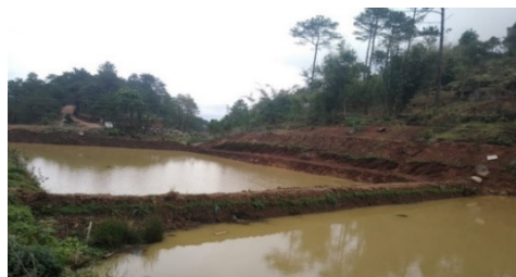
Community Tank at Mawkamoit, WKH with no RCC structure & micro irrigation.
