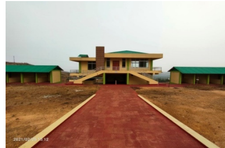
LBM at Pynursla, East Khasi Hills due to pending electric and water supply.
